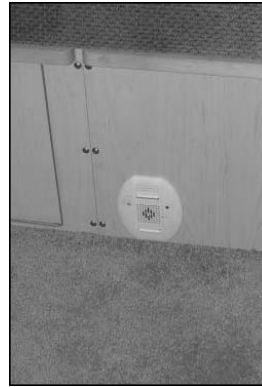
Picture F-P1: L.P.G. leak detector, Popular model.
